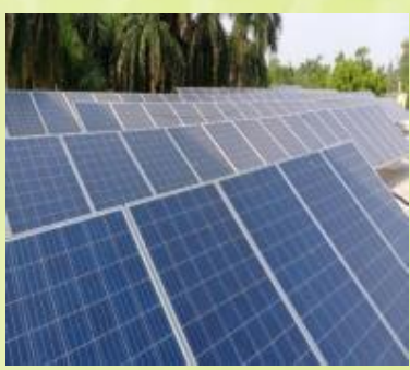
Roof of Central Canteen
