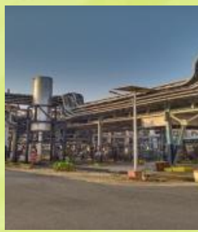
Solar Unit at Plant
