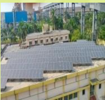
Roof of Control Room
