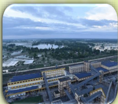
Bagging Top Floor
